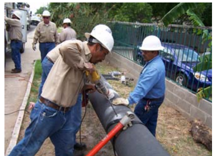
Field hole drilling
